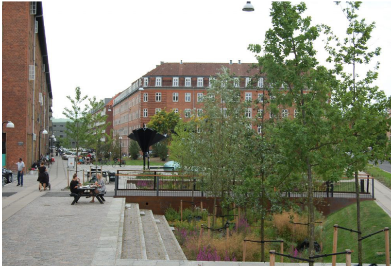
SuDS (Drainage Basin) in Tåsinge Plads by GHB Landscape Architects
