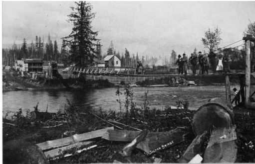
Sultan City Suspension Bridge
