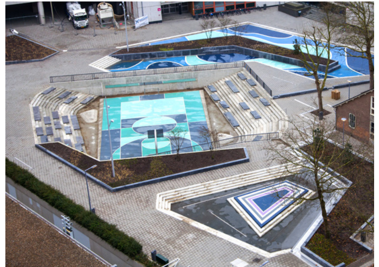
Water Drainage Square in Rotterdam by De Urbanisten
